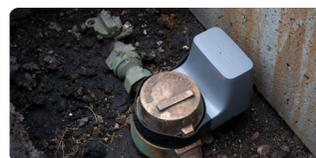
The Flowie-O water flow sensor uploads water flow data to the AlertAQ™ water intelligence platform for analysis and instant alerts.
